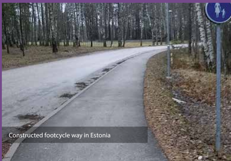
Footcycle way after reconstruction, Estonia
