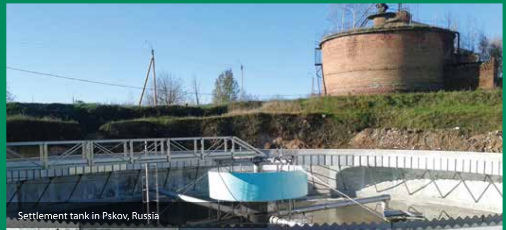
Electric and automatic devices in the wastewater treatment plant in Pskov, Russia
