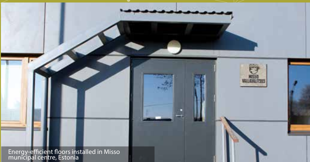
Misso municipality building after renovation
